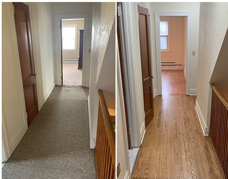
An upstairs hallway in the rectory is pictured before and after the Knights removed yards of carpeting and cleaned the wooden flooring
